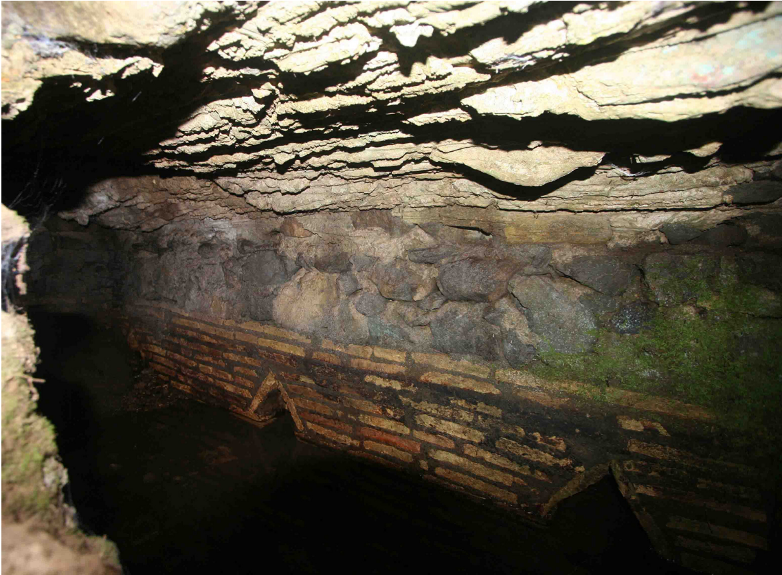
Fig. 17. Small spring chamber near Venticinque Vene (source of the twenty-five intakes), with three visible intakes, Grotte Renara. Photo: R. Taylor.
