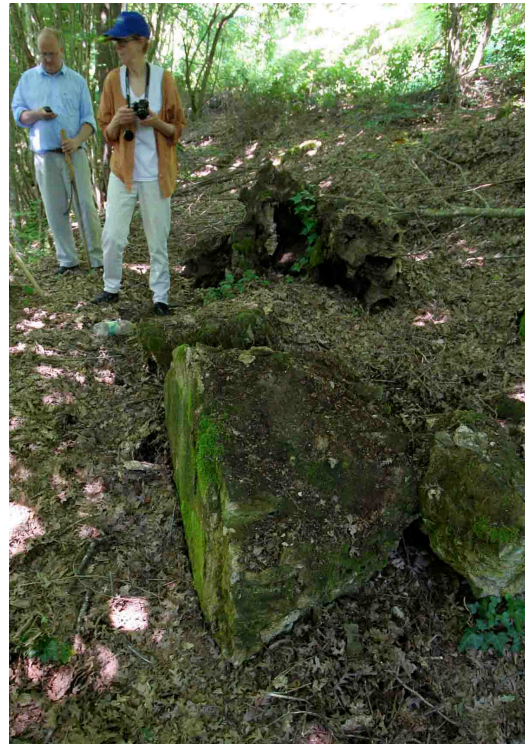
Fig. 29. Displaced chunk of opus reticulatum faced with opus signinum belonging to a side wall of the branch conduit of Santa Fiora in the Fosso della Fiora. Photo: R. Taylor.
