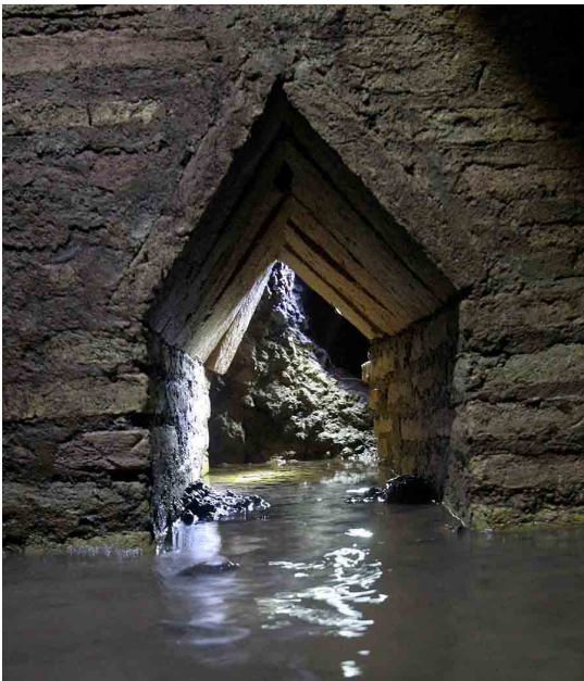
Fig. 21. Detail of an intake at the springhouse of Venticinque Vene. Photo: R. Taylor.
