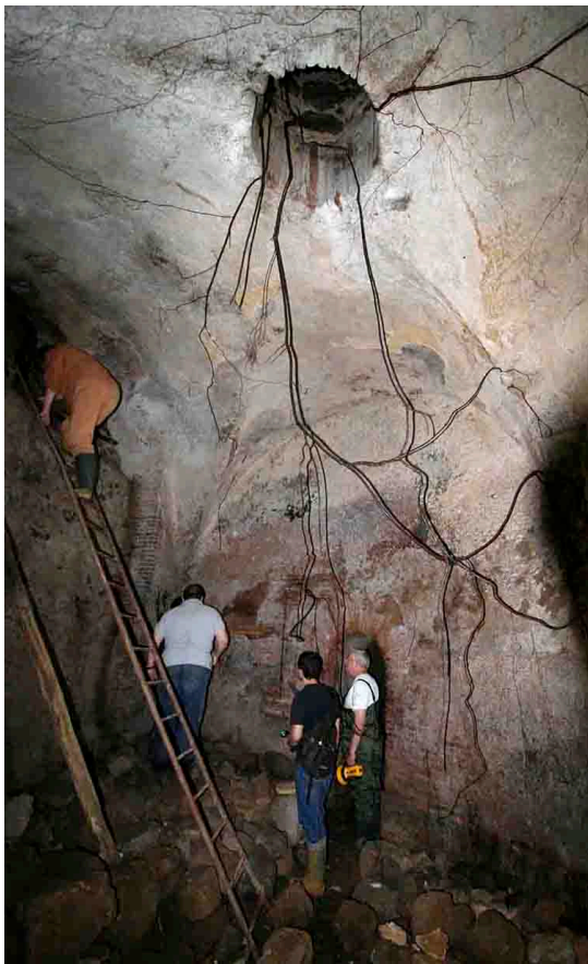
Fig. 2. Springhouse of Santa Fiora. The arched intake gallery can be seen below the oculus in the vault. Photo: R. Taylor.
