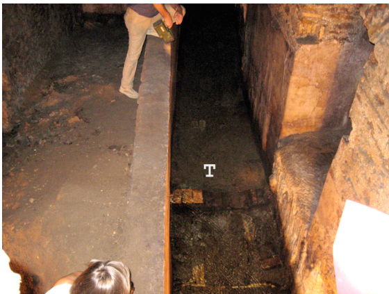
Figure 5. The remains of the small dam (T) built inside the channel of the Acqua Vergine. Leonardo Lombardi.
