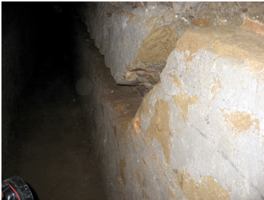
Figure 16. The remains of the channel in the sidewalls of the connecting tunnel. Leonardo Lombardi.
