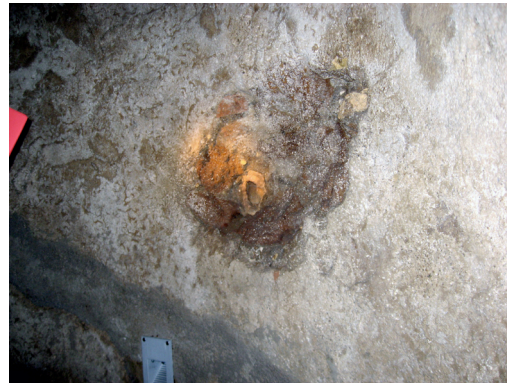
Figure 11. Remains of a tube embedded in the wall. Leonardo Lombardi
