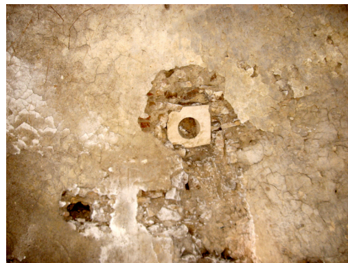
Figure 12. The remains of the stone slab found in the vault of the staircase chamber. Leonardo Lombardi.
