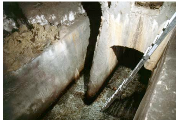
Figure 6. Remains of the second channel constructed parallel to the Acqua Vergine. Leonardo Lombardi.
