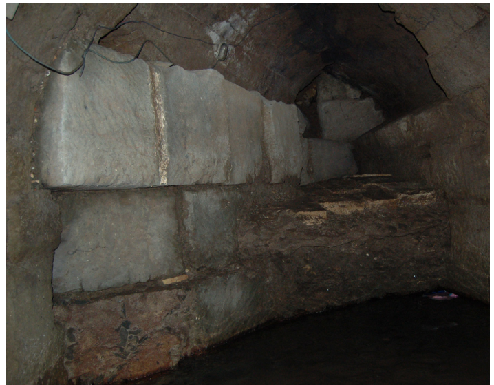
FIG. 7. Cloaca Maxima. Augustan Track. Domitianic closure wall at corner of Temple of Minerva. Photograph by John N. N. Hopkins
