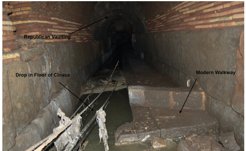
FIG. 9. Cloaca Maxima. Juncture of Flavian and Republican tracks. Photograph by John N. N. Hopkins
