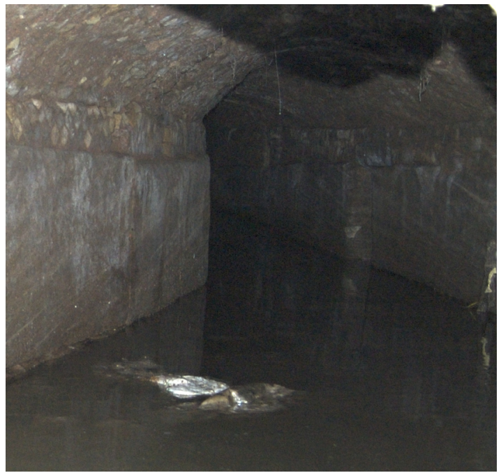
FIG. 14. Cloaca Maxima. Archaic track with later vaulting. Photograph by John N. N. Hopkins
